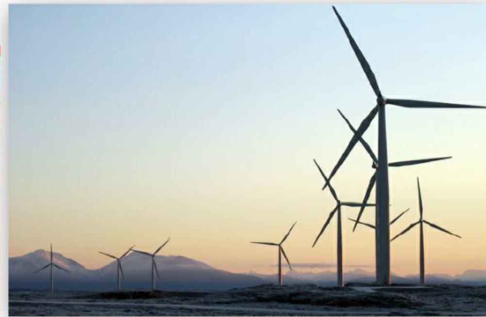
Wind farm at Smøla. Photo: Statkraft
