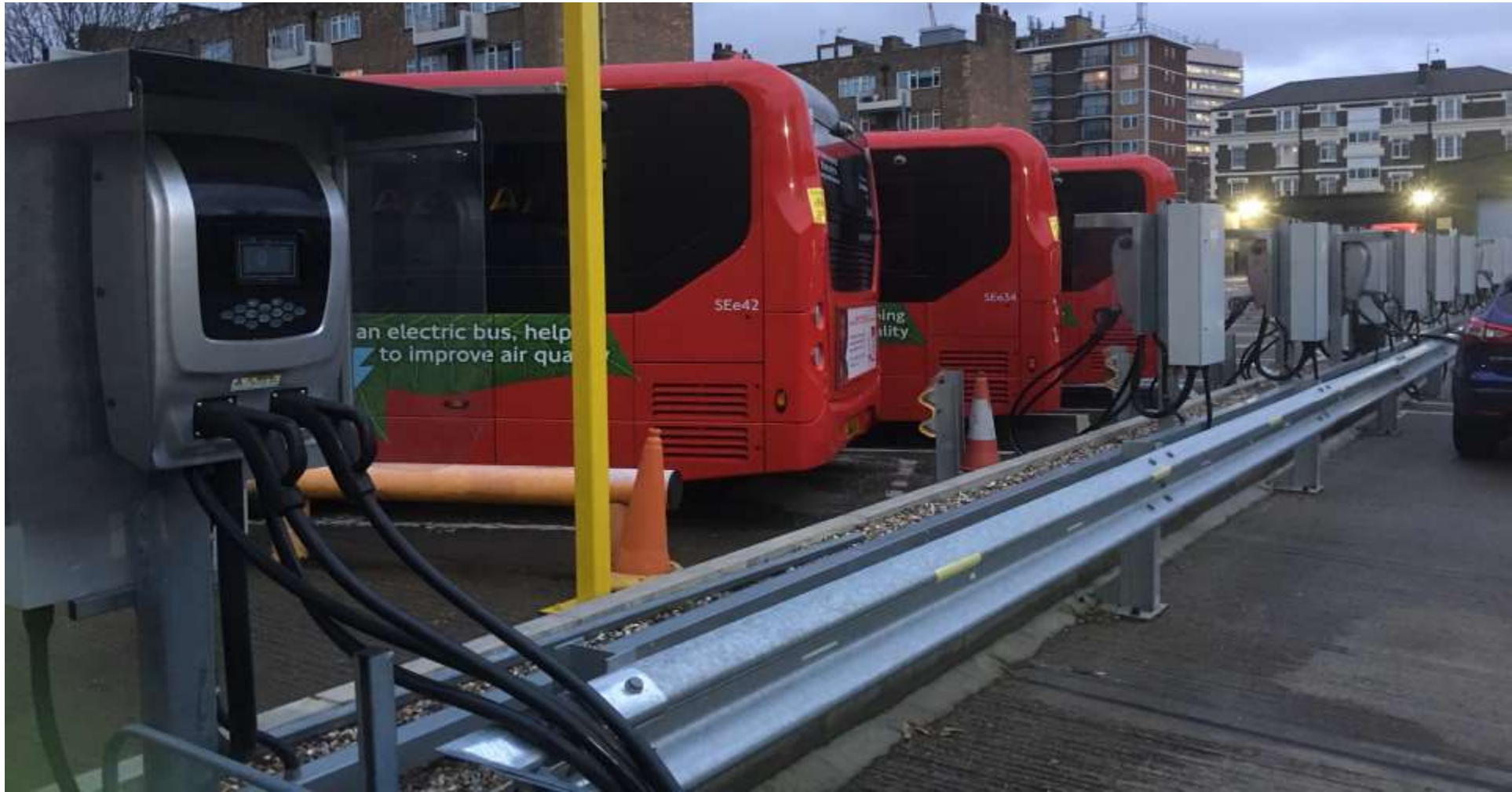
Waterloo, London bus garage: 46 electric buses smart charged overnight
