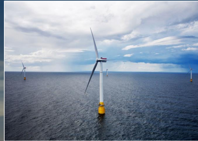
Hywind (2017 - Scotland) 5 x 6MW floating turbines
