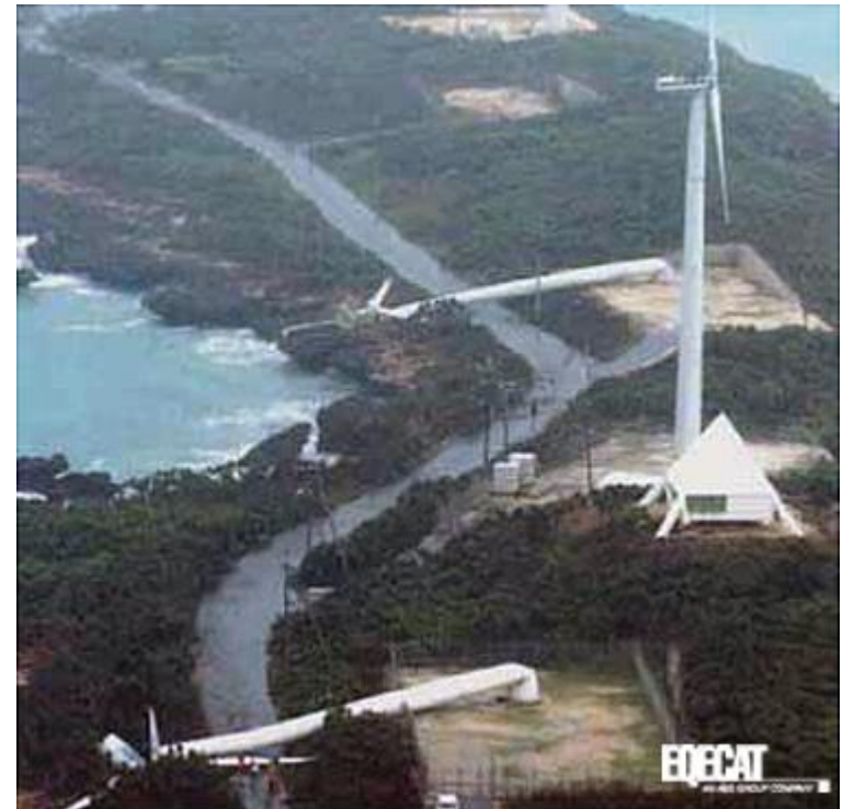
Damaged Wind Turbines from Typhoon Maemi, Japan 2003
